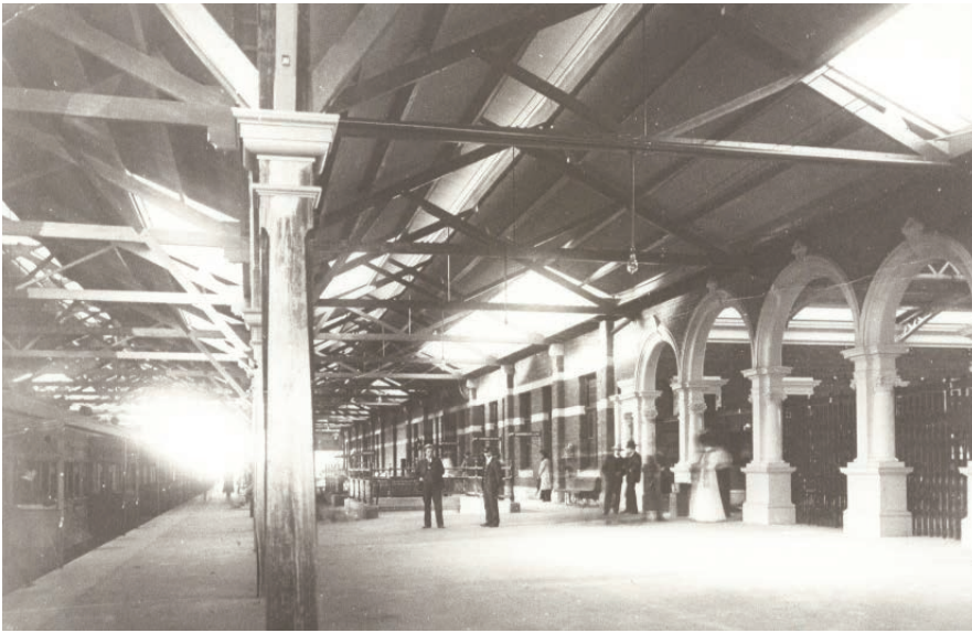
Above: Rare interior photograph c1920 showing subway to second platform (Courtesy Fremantle Local History Collection)
